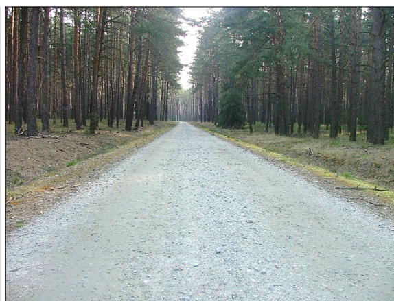
Fig. 2. View of the test road section with a crushed-stone surface (photo: S. M. Grajewski)
